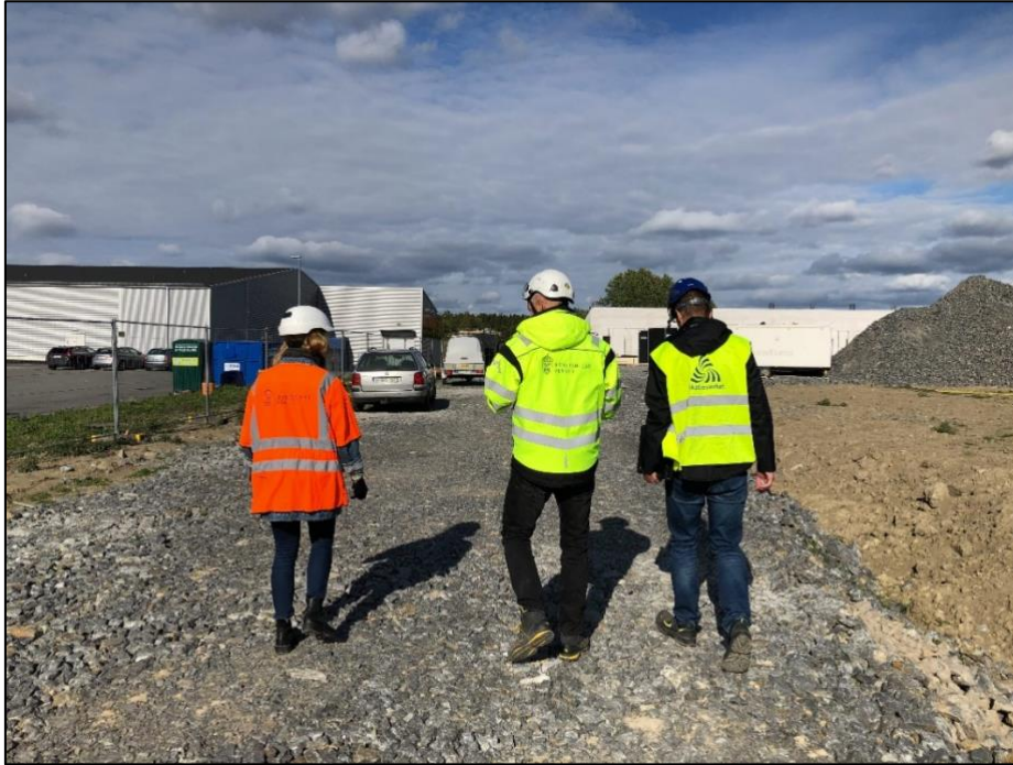
Photo 2. Inter-agency inspection of workplace in an industrial area.
